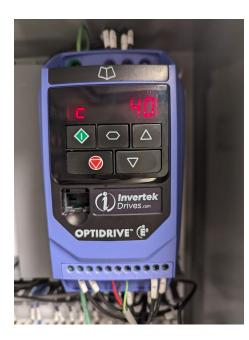
Invertek VFD - Press the Octagon to scroll through
